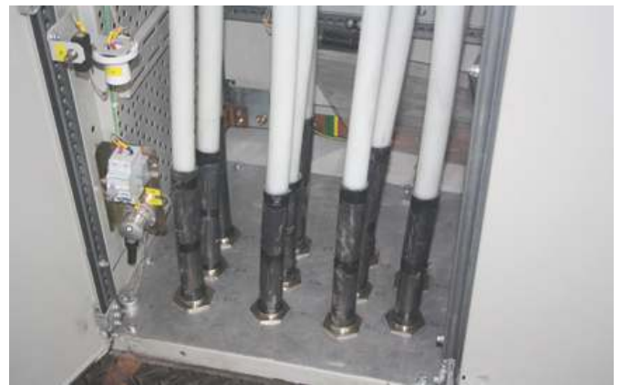
Figure 26 - Power cable terminals bottom cable entry
