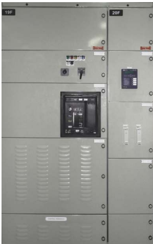
Figure 1 - Typical PCC panel
