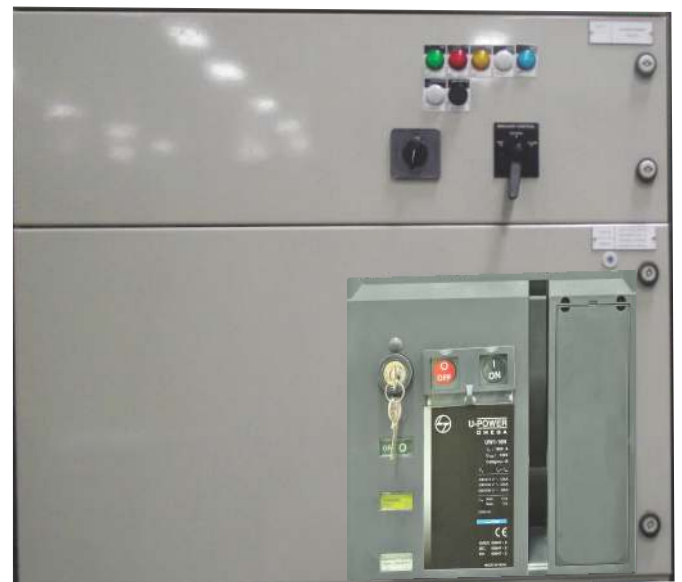
Figure 35 - Front facia of ACB
