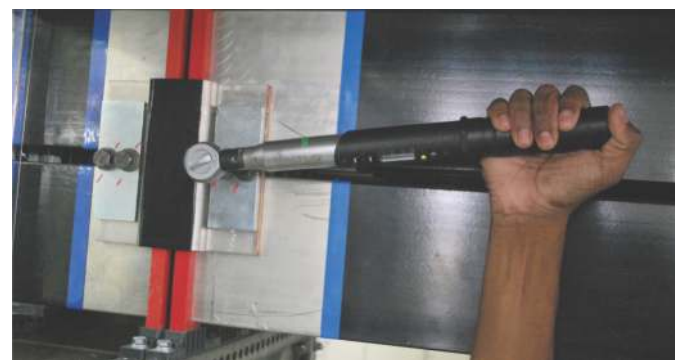
Figure 19 - Tightning of Busbar joints
