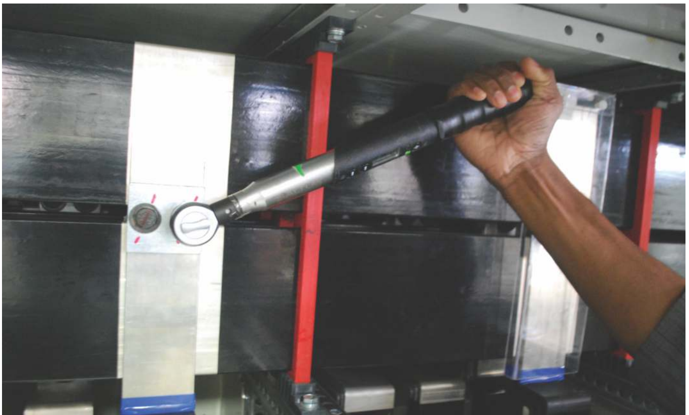
Figure 36 - Tightening of Busbar & Dropper Joint
