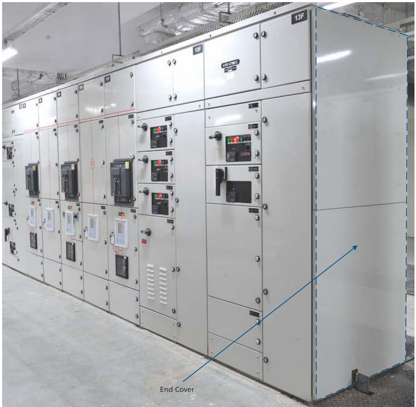
Figure 34 - Extension of Panel
