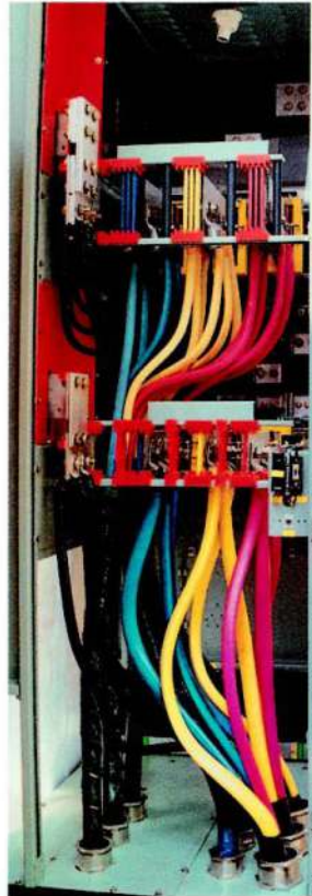
Shrouded linkwork ensures complete safety in cable alley.
