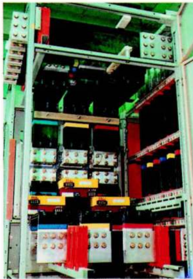
Interlaced link work for buscoupler
