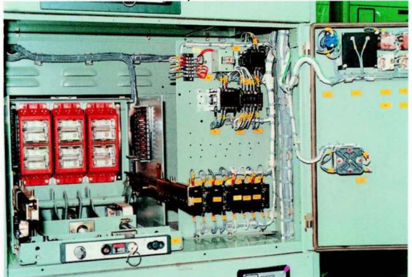
ACB cradle with spring loaded safety shutters and telescopic rails. Auxiliary equipment can be mounted in same compartment.
