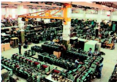
Air Circuit Breaker assembly shop.
