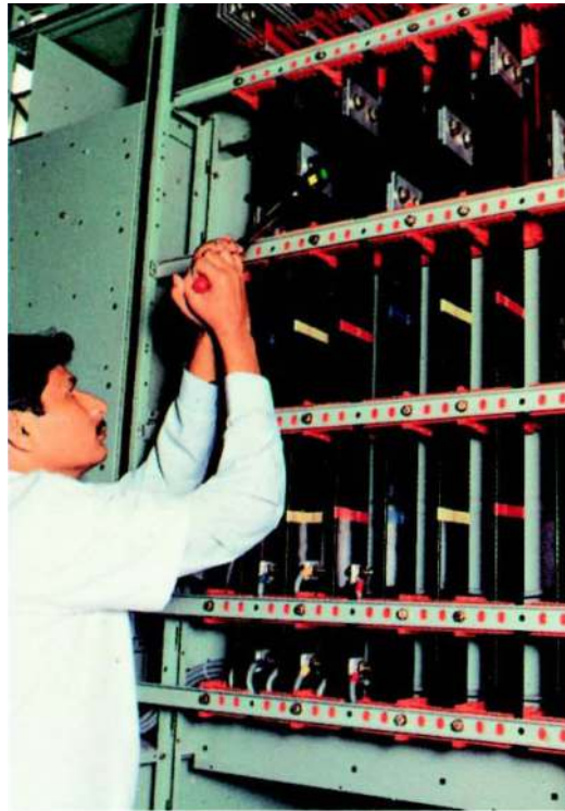
Stage inspection during assembly ensures reliability.
