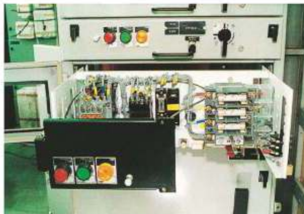
200 mm module in maintenance position
