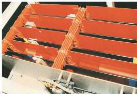
Interphase barriers for horizontal busbars
