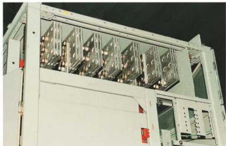
Interleaved arrangement of busbars
