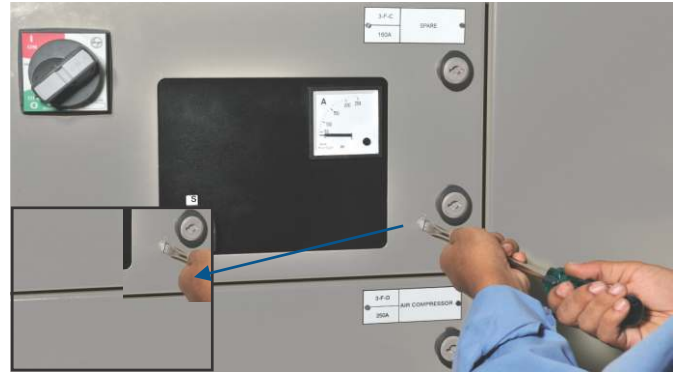
Figure 17 - Door defeat interlock
