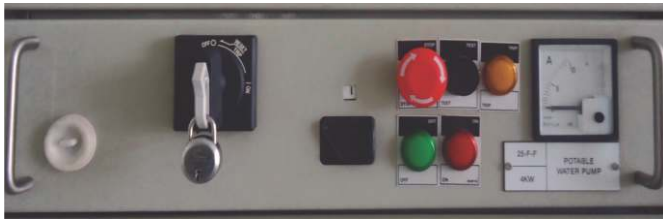
Figure 14 - Full width power switch padlocking
