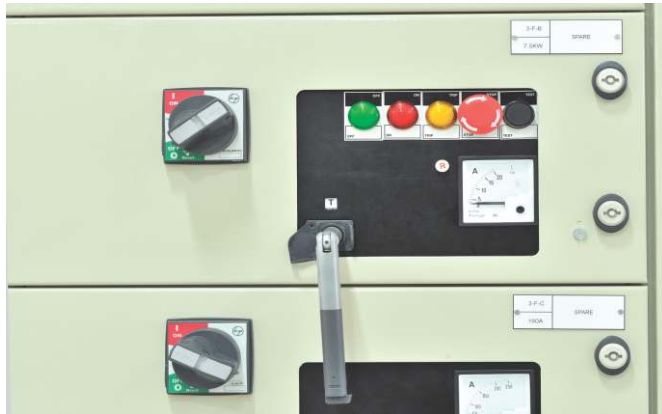
Figure 55 - Full width module in Test position
