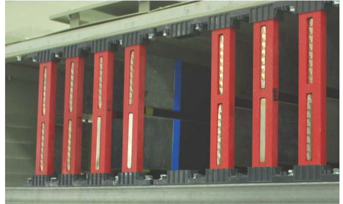
Figure 3 - Double Deck Arrangement of busbars
