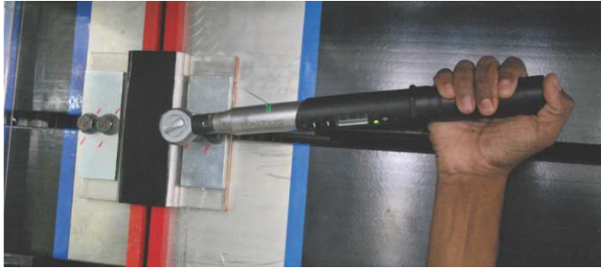
Figure 39 - Tightening of Busbar joints
