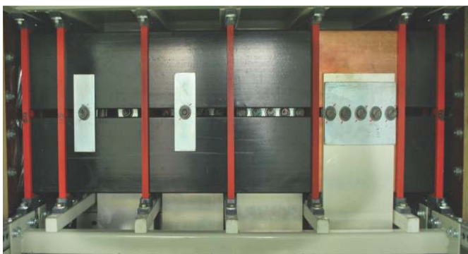
Figure 59 - Tightening of Busbar & Dropper Joint
