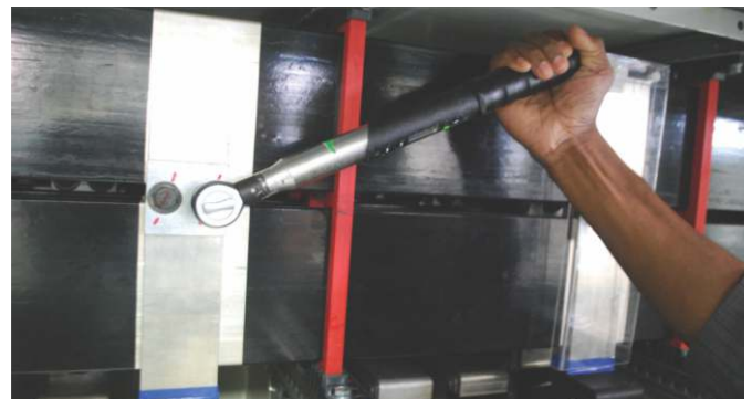
Figure 60 - Tightening of Busbar Joints
