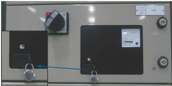
Figure 15 - Full width module padlocking
